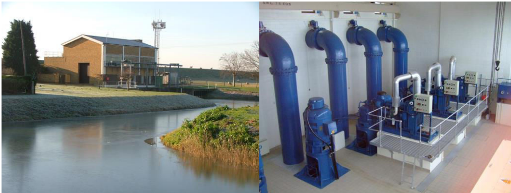
Figures 7-10 and 7-11: Cross Guns Pumping Station inside (left) and outside (right). Source: North Level District IDB
