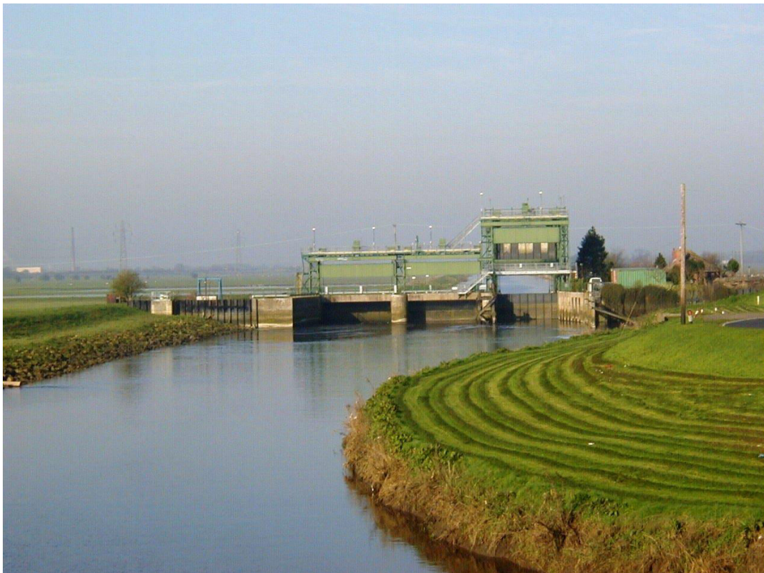
Figure 7-3: Dog in the Doublet sluice when the tide is not so high. Source: Environment Agency.
